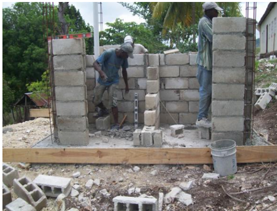
PHOTO 8: CONSTRUCTION BLOC LATRINES
